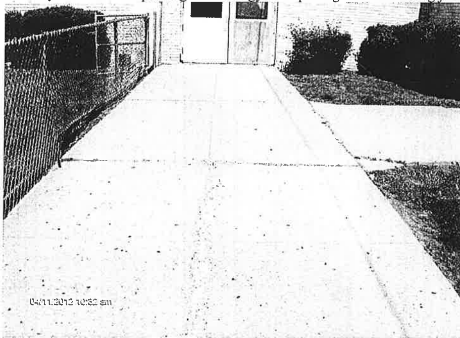
Walkway From Rear Parking Lot To Gym
